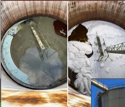
Analysis of the collapse of the floating roof of a storage tank
